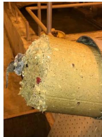
Image 1: A mound of wipes pulled out of a sewage pumping station after a blockage was discovered.
